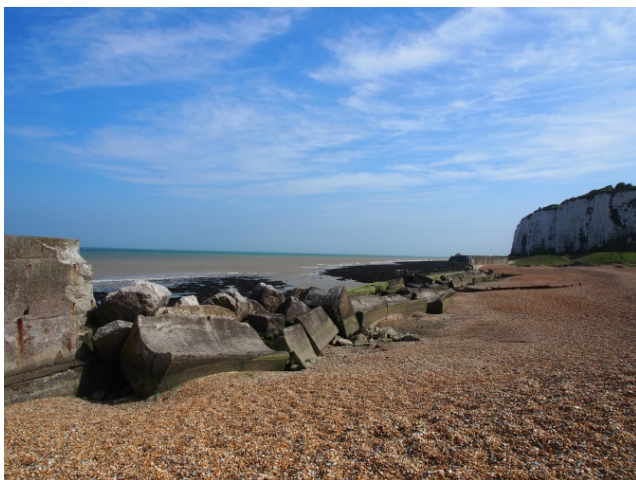
Seawall toppled by storm, Kingsdown
