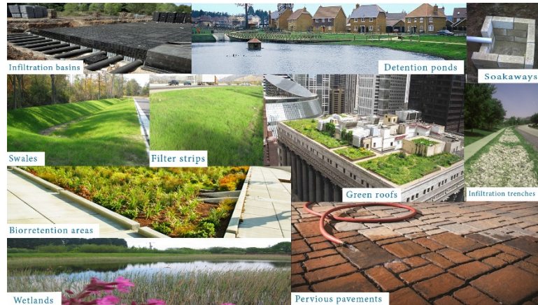
Figure 12 Examples of Sustainable Drainage Systems used in urban developments to prevent flash flooding and erosion as well as treatment of water before it enters watercourses (Hydrologia Sostenibile, 2020)
