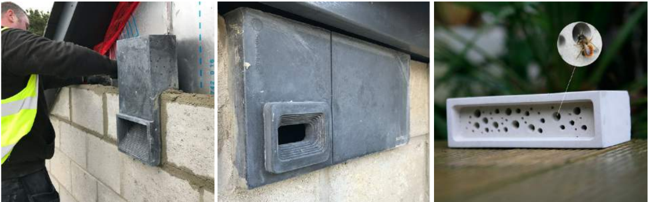
Figure 7. Building bricks tailored to provide habitat for microbats, birds (swifts) and solitary bees 13
