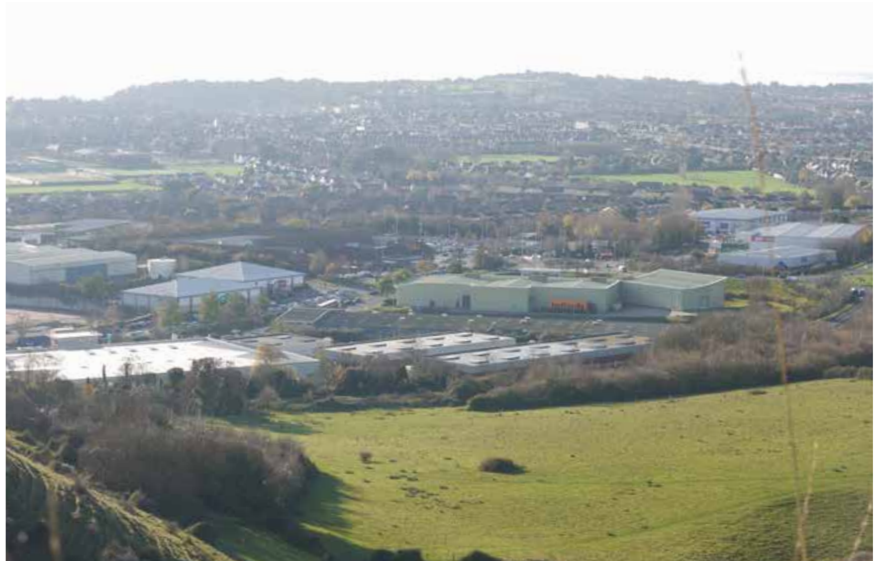
Highly reflective roofing material
